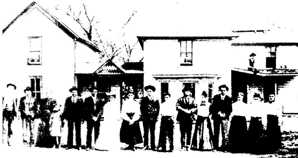
The Rucker Hotel was on the northwest corner of Second Street and Broadway. Built by W. F. Rucker about the turn of the century, the hotel burned about 1912 or 1913. Pictured from left to right: ...?..., 2. W. F. Rucker, 3. Mary E. Rucker, 4. Florence Rucker, 5. Vernie Harper, 6. ...?..., 7. ...?..., 8. Nan Rucker, 9. ...?..., 10. ...?..., 11. Elliot Rucker, 12. ...?..., 13. ...?..., 14. ...?..., 15. Anna Lee Rucker, 16. ...?.... The young boy on the porch roof is Robert Clyde Smith, grandson of W. F. and Mary E. Rucker.
