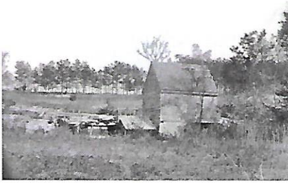
Mechanicsville, Virginia - Ellerson's Mill
